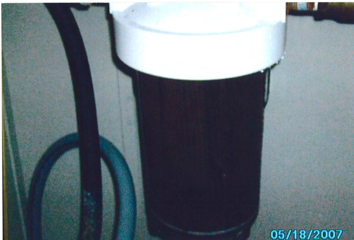
Photo 6: May 18, 2007 – Water filter in Complainant's home after less than two months
