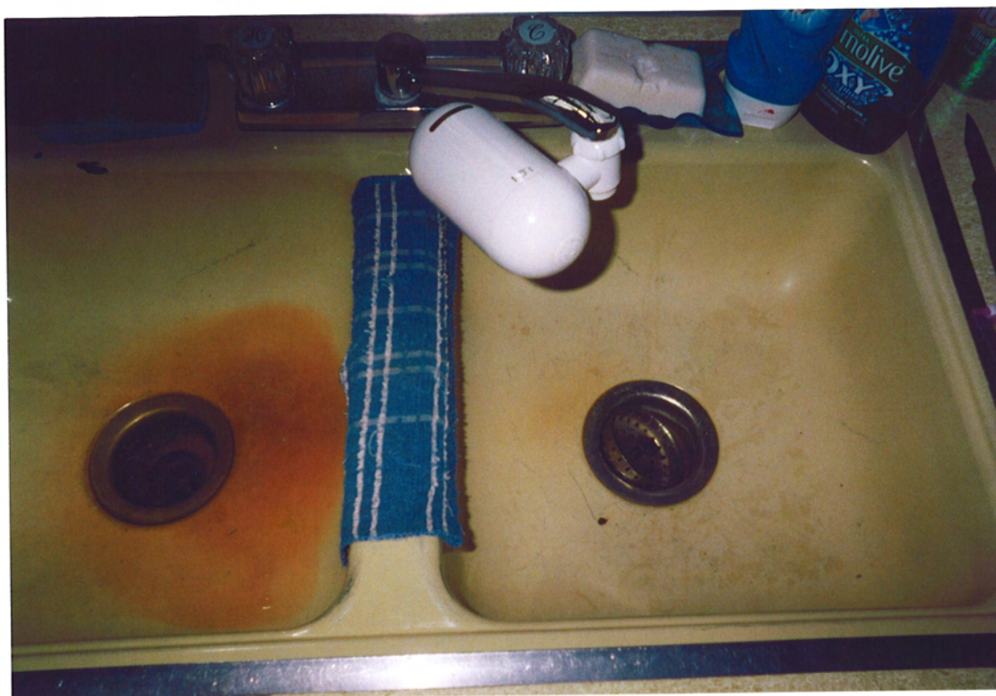
Photo 11: Complainant's kitchen sink stains and tap filter
